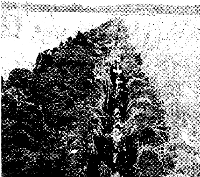
One of the drainage tile lines dug up. The dirt is pushed back in with the bottom of the layer going in first and then the top soil. This field may change from a mesic to wet-mesic prairie restoration.
