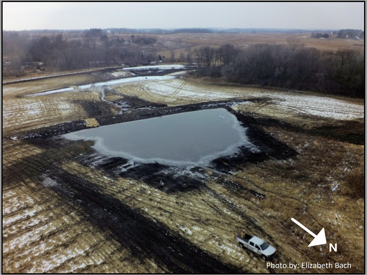
Photo 5: Drone picture showing the newly constructed dykes and where the drain tiles were removed
