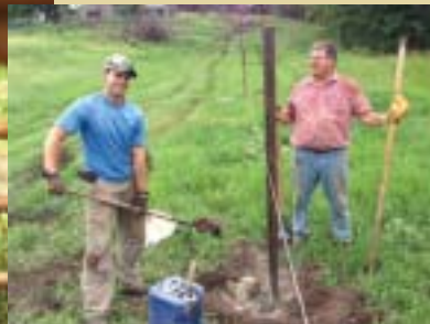
CODY CONSIDINE AND MIKE CARR, BUILDING FENCE ★
